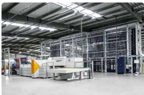
Automated bending centre - research and development hall
